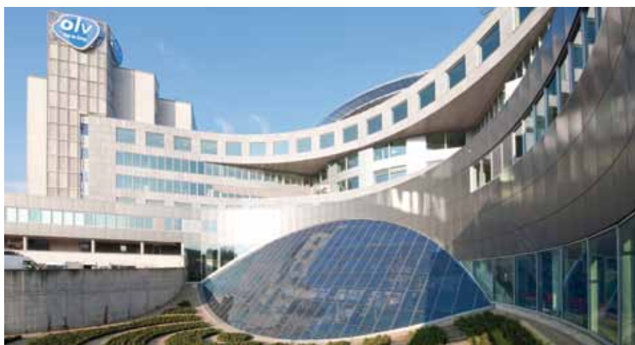
The General Hospital OLV Aalst in Belgium, designed by VK Studio
