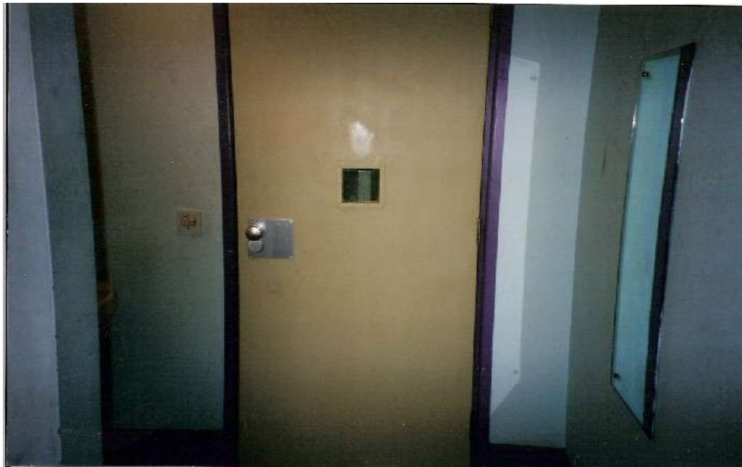
Small Health. Watch panel window on ward's bedroom doors.
